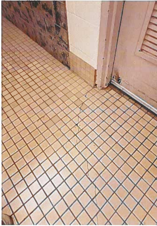
Photograph 3: Bath House - Floor Tile Crack
