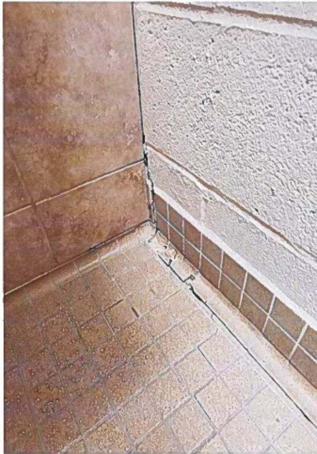
Photograph 4: Bath House - Floor Tile Damage
