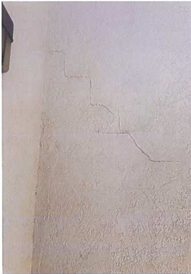
Photograph 5: Bath House - Stepping Crack in Exterior Wall
