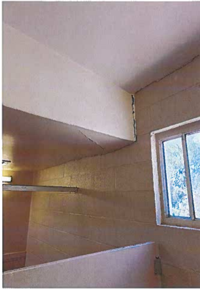
Photograph 1: Bath House - Ceiling and Wall Separation
