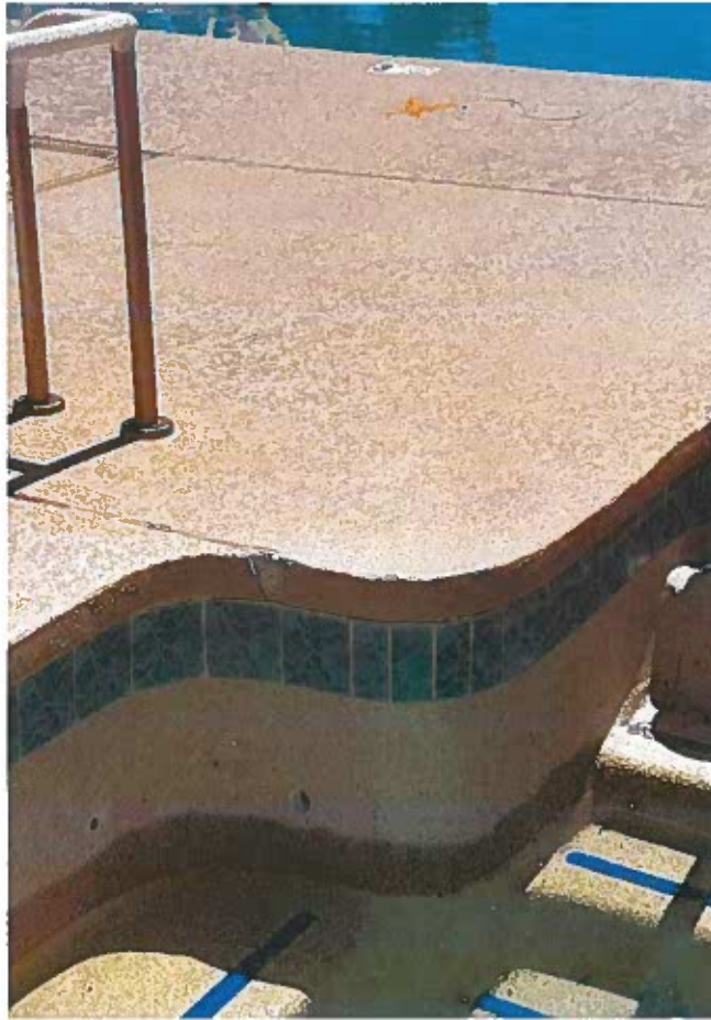
Photograph 11: Spa - Deck Separation
