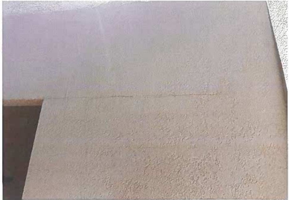
Photograph 6: Bath House - Horizontal Crack in Exterior Wall
