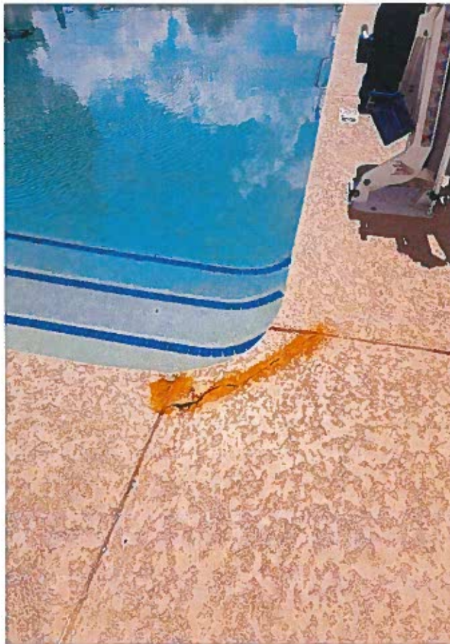
Photograph 7: Concrete Deck - Corner Crack
