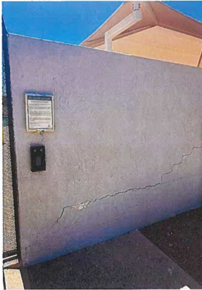
Photograph 12: Equipment Area - Horizontal Crack in Masonry Wall
